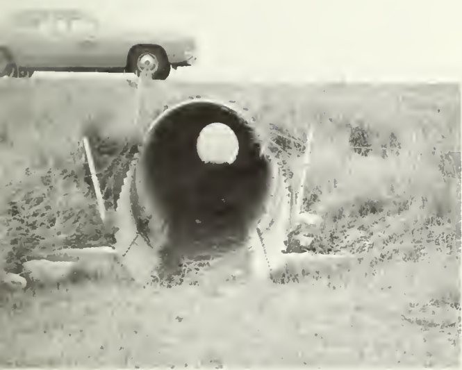
EAST ENTRANCE Note concrete stabilization
